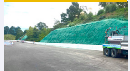
Completed Flexterra HP-FGM application
